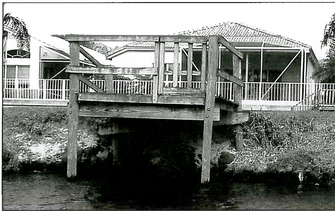
The Hillsboro Canal's right-of-way extends 40 feet or more landward from the top of the bank. The placement of encroachments such as a boat dock have caused the bank slope to erode or become detached and fall into the canal.
