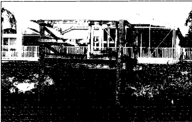
The Hillsboro Canal's right-of-way extends several feet landward from the top of the bank. The placement of encroachments such as a boat dock have caused the bank slope to erode or become detached and fall into the canal.
